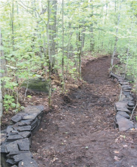
Rocks removed during trail construction line a portion of the Turtle Lake Trail
