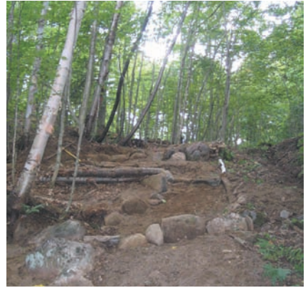
Steps are added on steep inclines for safety
